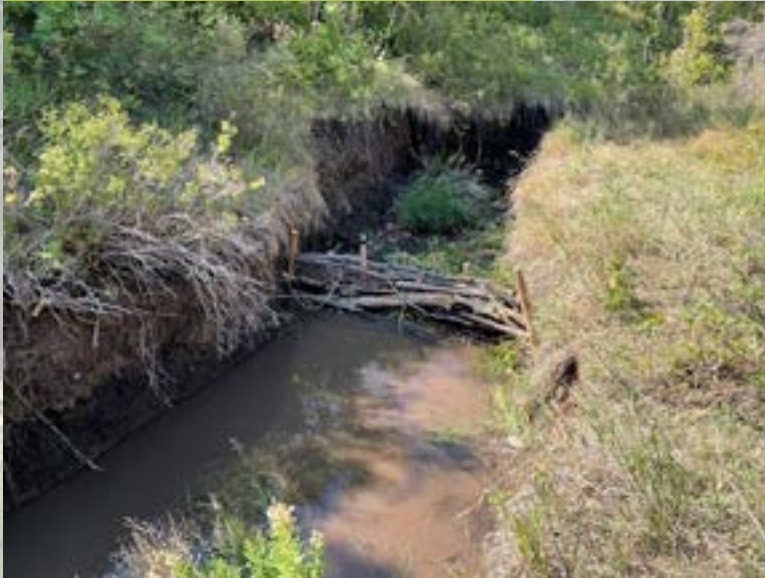
Volunteers coordinated by Sageland Collaborative installed this beaver dam analogue in Parleys Creek. September 2024
