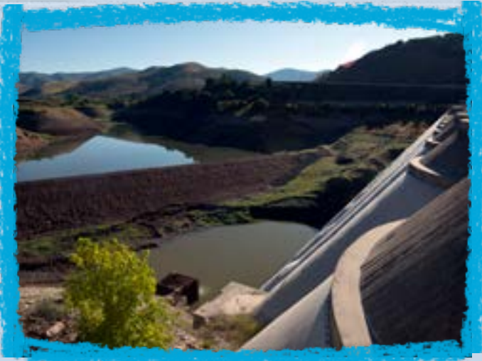
Infrastructure improvements at Mountain Dell Dam ensure efficiency at Parleys Water Treatment Plant September 2023
