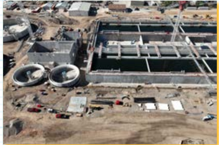
A sitewide view of progress at the New WRF October 2024
