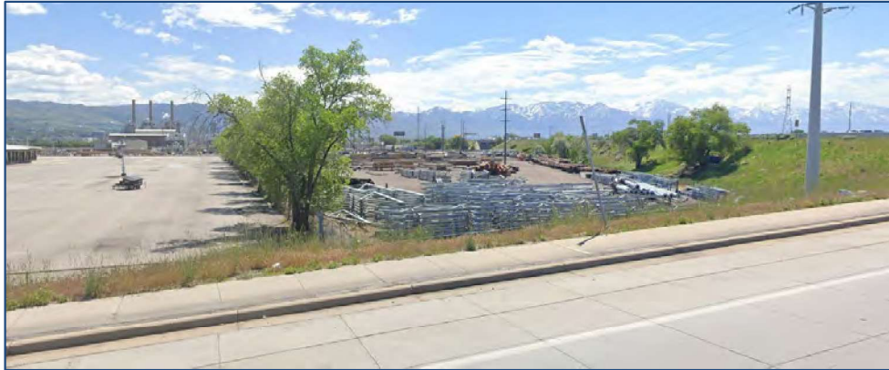
Subject property along Redwood Road and offramp from I-80
