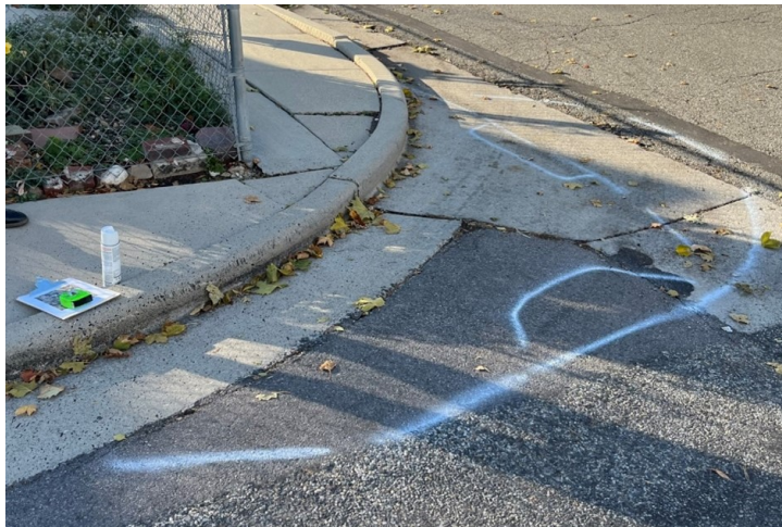
Potential layout for new curb ramp and sidewalk at 200 East and Downington Ave.
