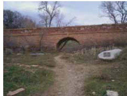
Photo 24: Sandstone aqueduct and interpretive monument.
