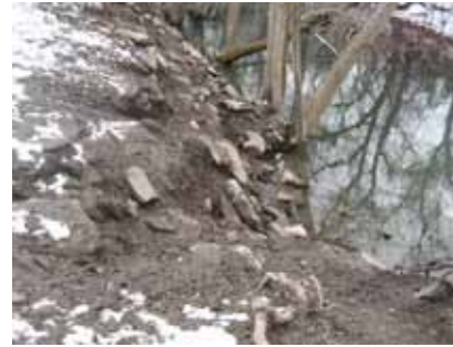
Photo 9: Erosion caused by high-traffic human and dog access to the creek.
