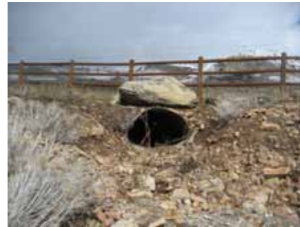
Photo 14: Outlet of third 48" Culvert.
