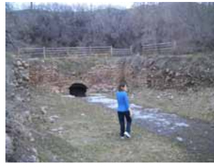
Photo 22: Dudler's Inn cellar and foundation.
