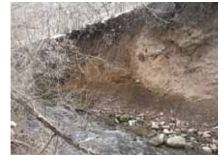
Photo 8: High erosion potential of a vertical bank.
