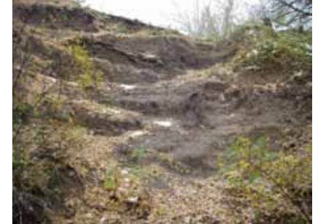
Photo 19: Bank erosion adding sediment to the creek.
