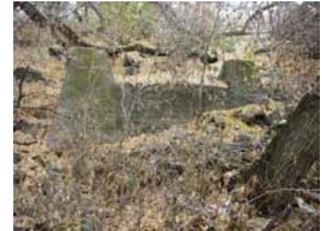
Photo 25: Remnant foundation from gravel and concrete operations.
