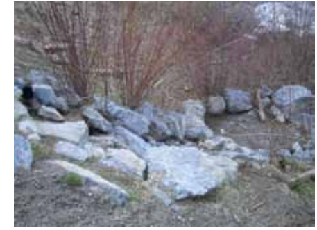
Photo 13: Outlet of Mary's Spring through culvert 2.
