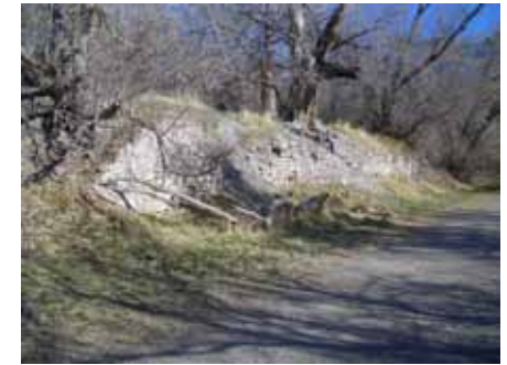
Photo 23: Rock wall lining the historic road.
