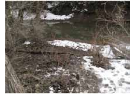
Photo 10: Erosion caused by high-traffic access to creek and storm runoff.
