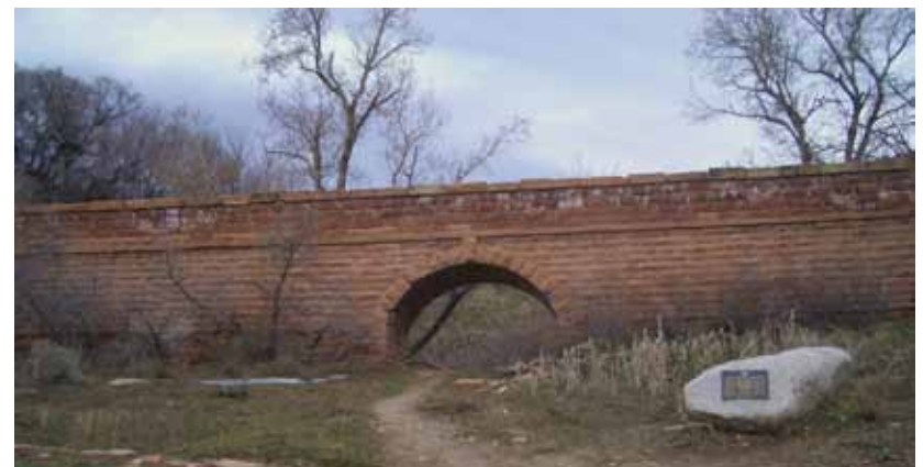
Sandstone aqueduct, a remnant from the historic Pleasant View Canal.
