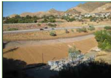
Photo 36: Parley's Trail and restoration area from its construction, next to I-80.
