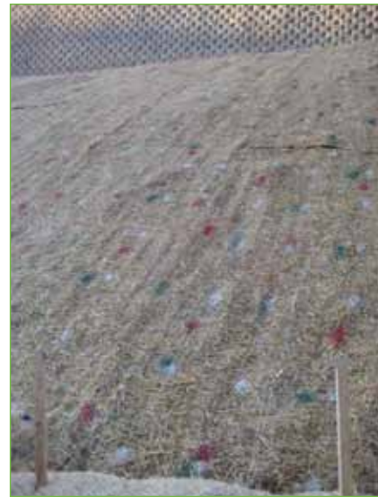
Photo 37: Erosion control blanket.
