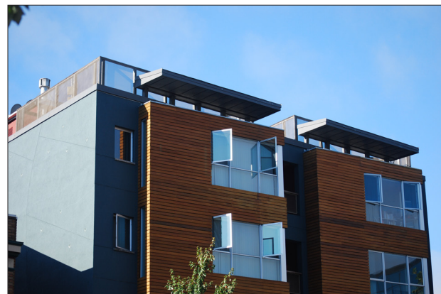
Recent apartment design creatively using traditional materials, resident open space and natural ventilation.
