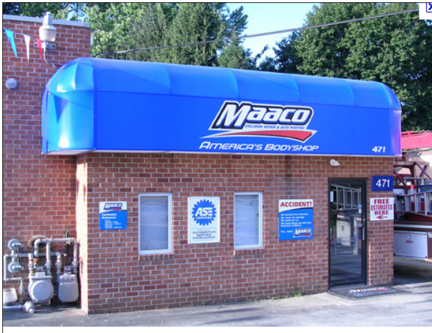
The materials and shape of this awning are discouraged.
