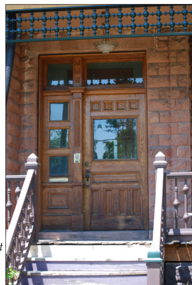
The decorative detail of the porch and balustrade complement this entrance and panelled doorway.
