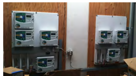
Irrigation Equipment - Automatic Controllers Source: Cemetery Planning Team
