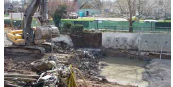
Ground water can have an impact on development. Often times, basements and subterranean parking structures are required to pump ground water to prevent it from damaging buildings.
