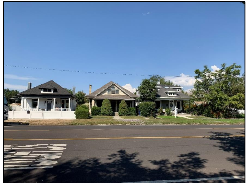
Existing single-family homes along 200 South – facing north
