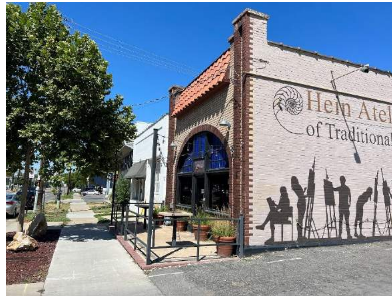
Building adjacent to project site to the east. White building is in the project site and is proposed to be demolished.
