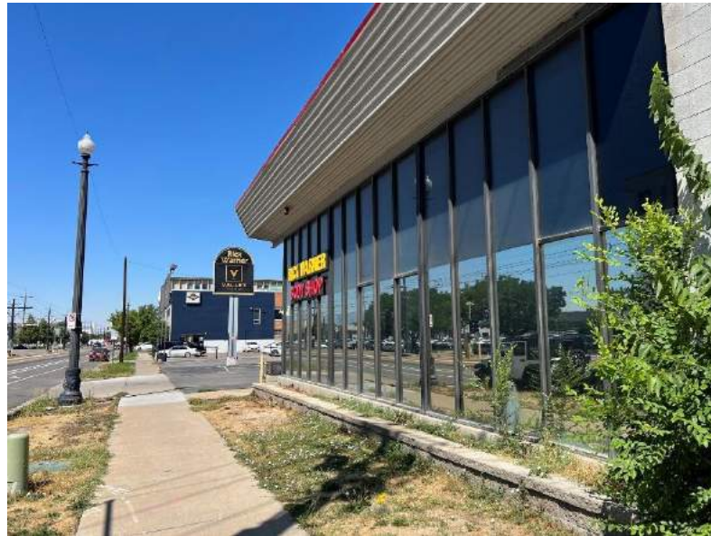
Project site looking west
