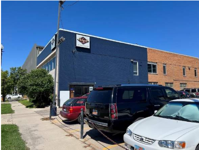
Project site. Blue building to be demolished. Gray building is adjacent to project site.
