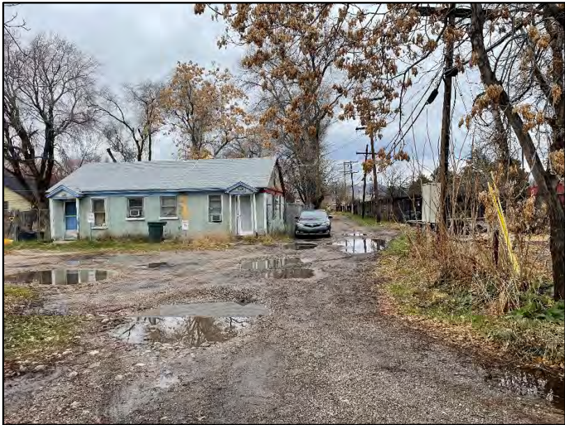
Alley to the west and duplex at the rear of 2027 S Richards
