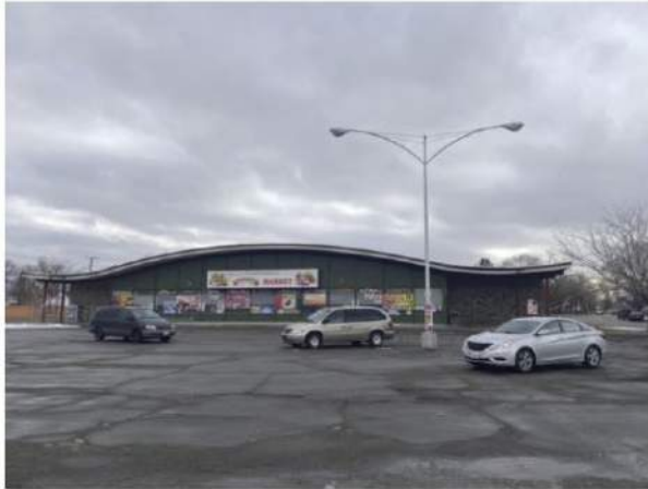
Front of Existing Building
