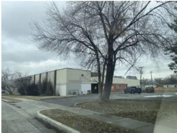
Back of Existing Building
