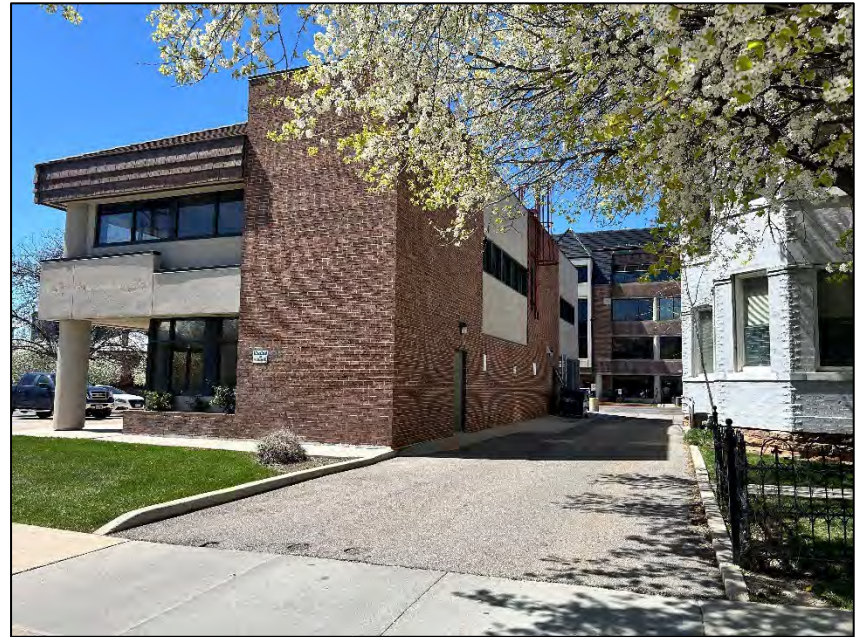
Subject Property 2 – Office building at 475 E 500 S – driveway access #1
