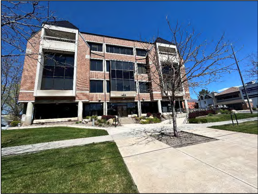
Subject Property 1 – AFCU building at 455 E 500 S
