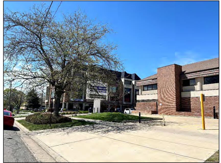
Driveway #3, which is closed and blocked with bollards
