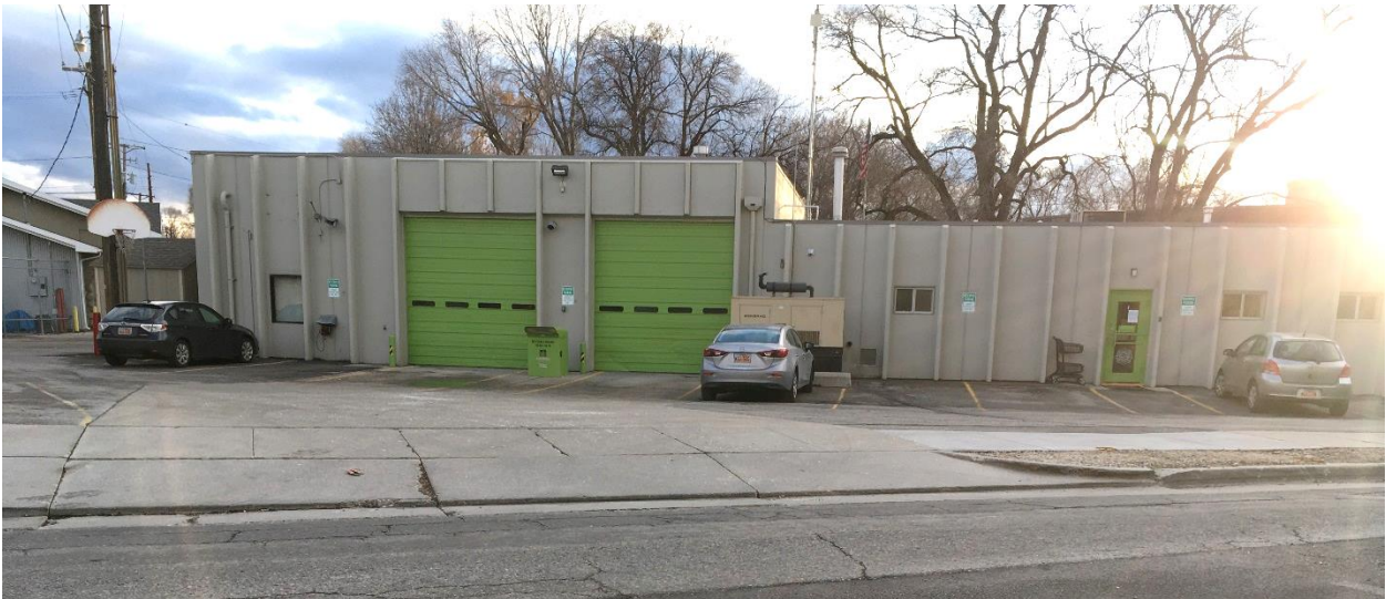
View of the north side of the site looking south from Sugarmont Drive, showing the back of the former Fire Station Building
