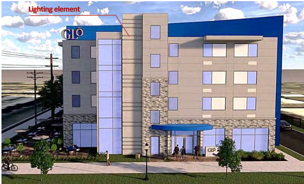
Image 10 – Rendering of the front façade of the building, where the lighting element with EIFS is most visible.
