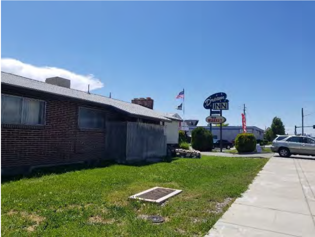
Image 9 – View of the existing hotel from the northeast corner of the lot on North Temple.
