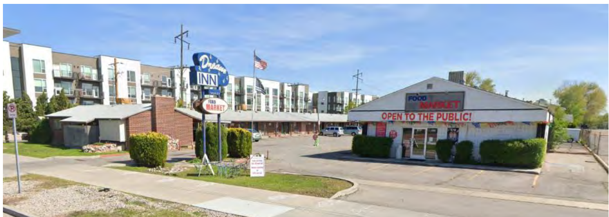
Image 6 – Existing buildings on site viewed from North Temple.
