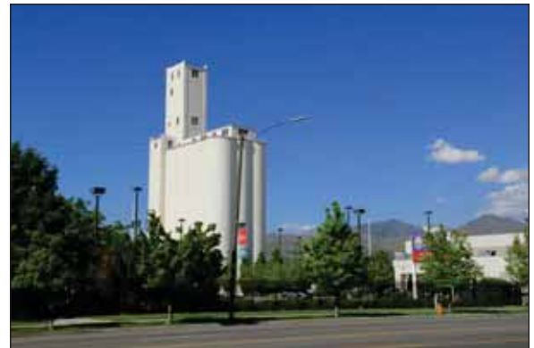
The grain silo at Welfare Square is the tallest structure in West Salt Lake and an easily identifiable landmark from the interstate.
