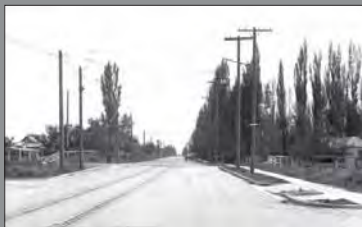
900 South & 900 West, Salt Lake City, circa 1917. Photo courtesy Utah State Historical Society
