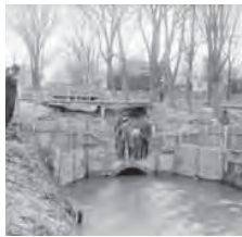
900 South canal pipe
