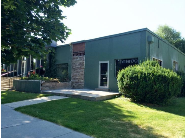
Front (North) View
