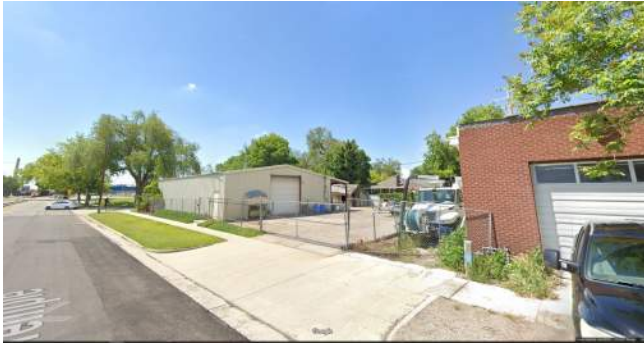
Looking North West at Site
