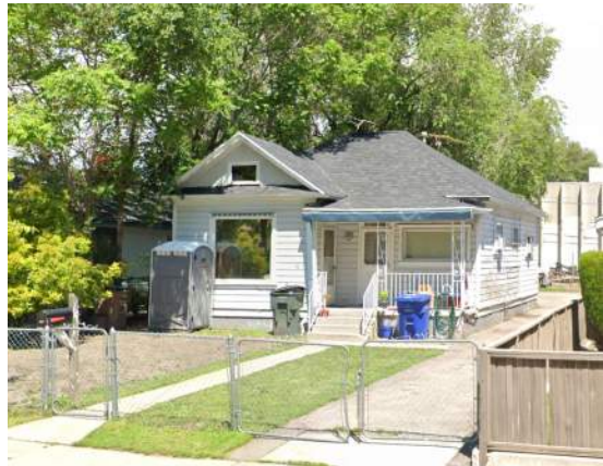
Existing Warehouse at 30 W Chicago St will be Removed
