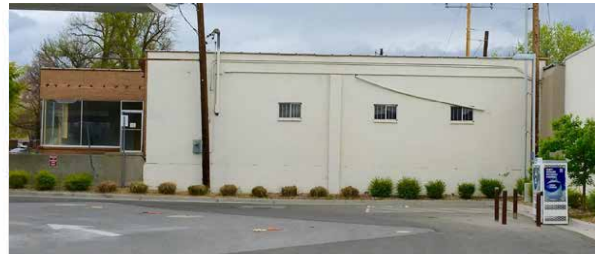
EXISTING SOUTH FACADE
