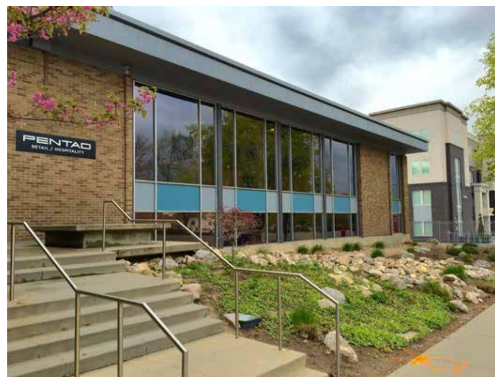
2 - OFFICE BUILDING: 560 E 500 S
