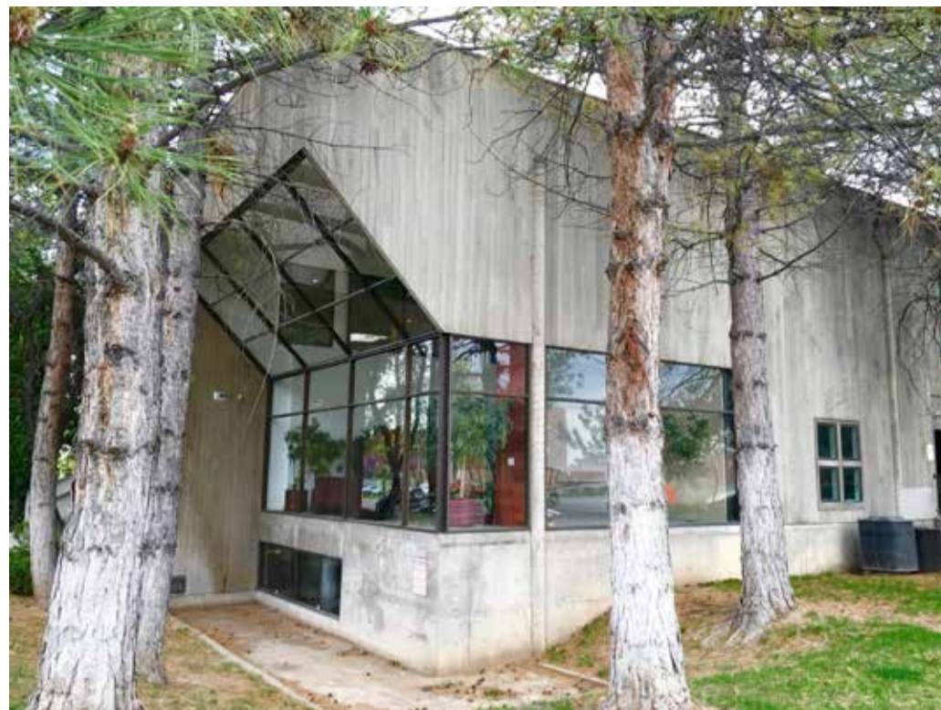
3 - OFFICE BUILDING: 510 S 600 W
