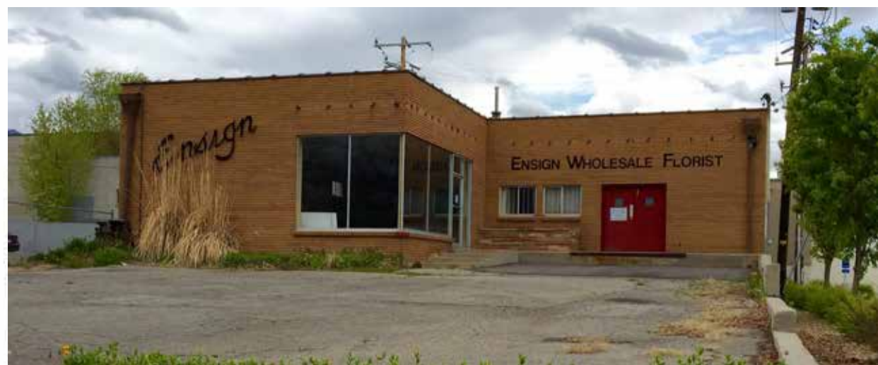
EXISTING WEST FACADE
