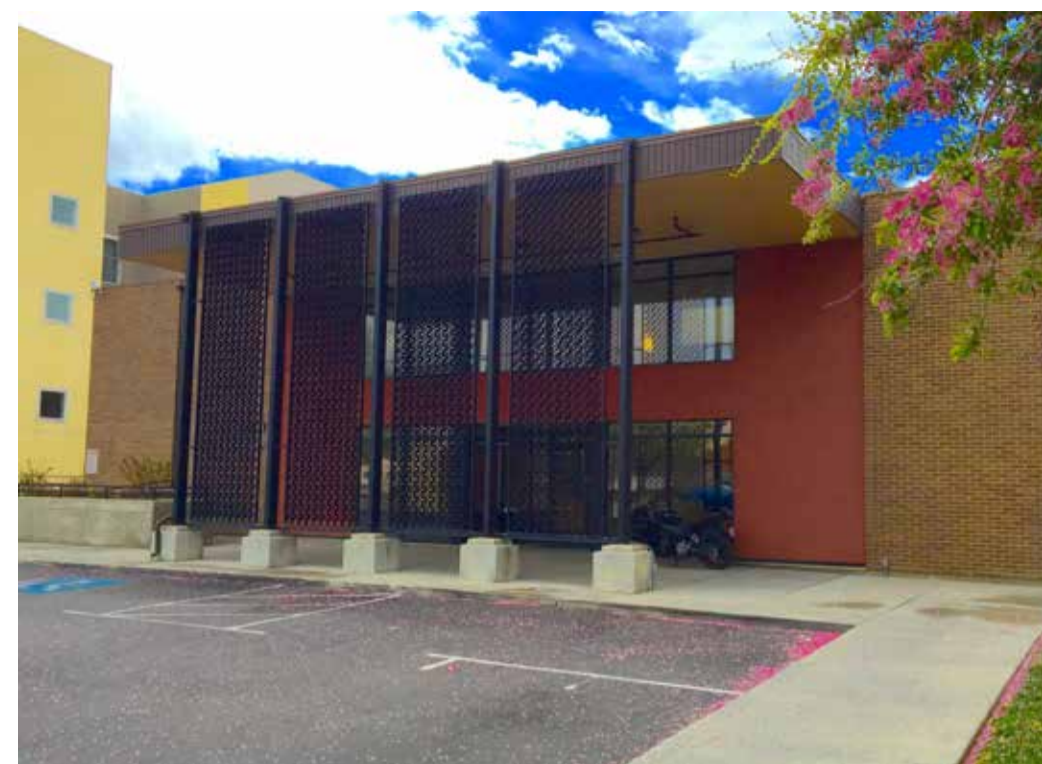
3 - OFFICE BUILDING: 530 E 500 S
