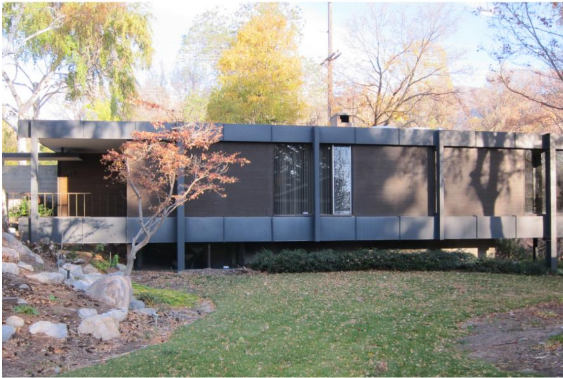
Photograph 3 of 18. View of Northeast elevation. Camera facing southwest.
