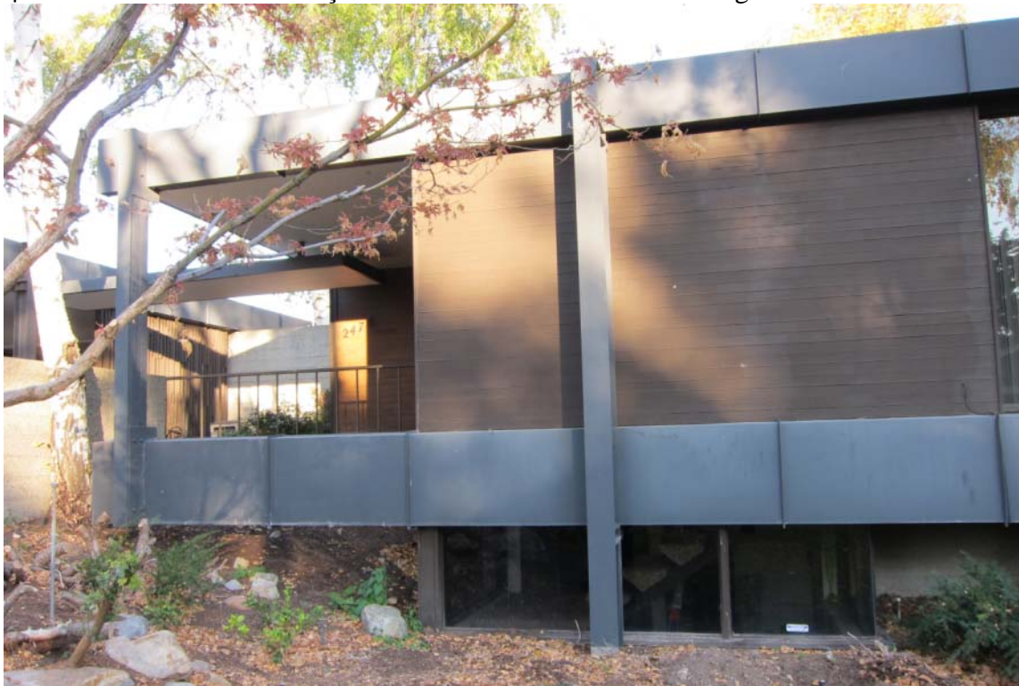
Photograph 8 of 18. Formal sitting area with built-in furniture. Camera facing east.
