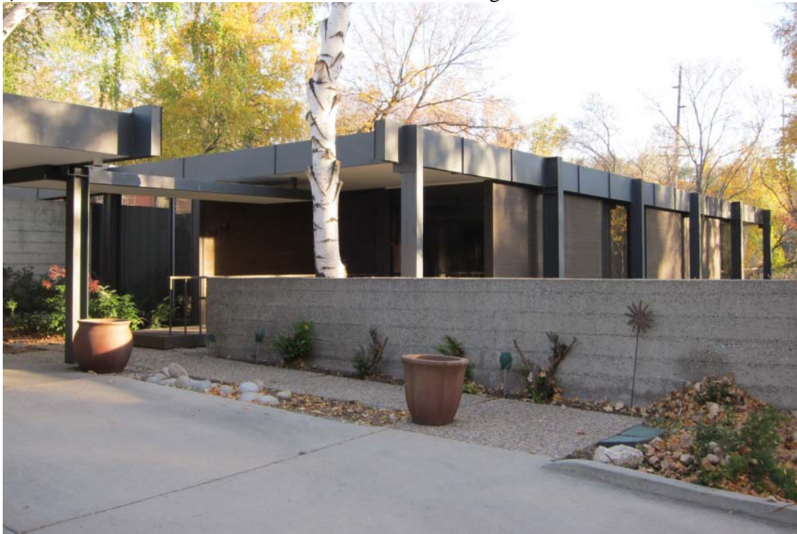
Photograph 1 of 18. View of Northwest elevation. Camera facing southeast.
