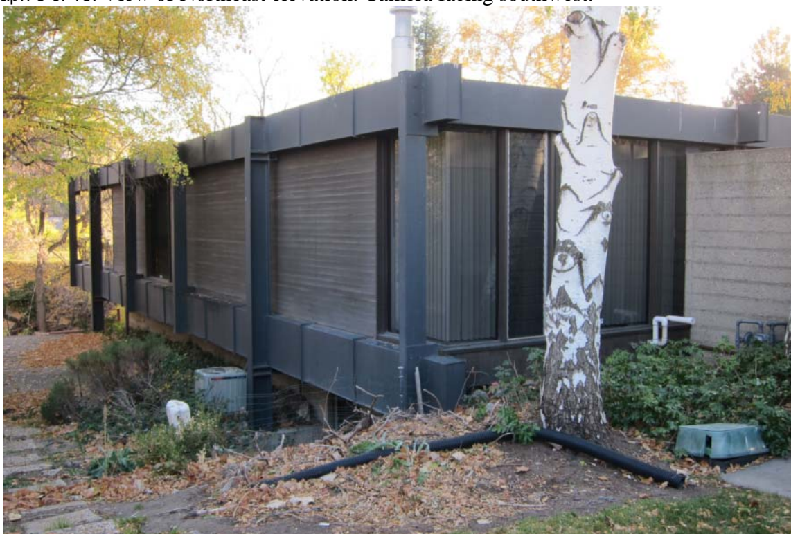
Photograph 4 of 18. View of South elevation. Camera facing north.
